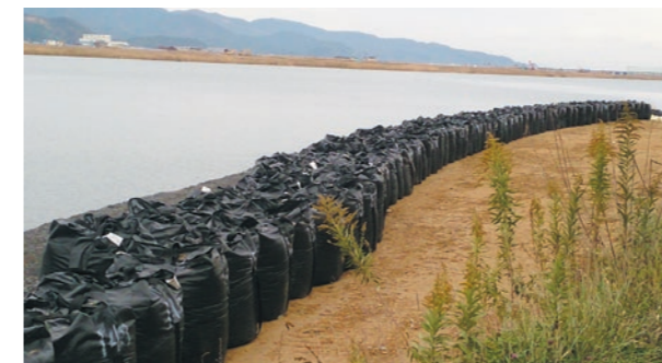
Large high-performance sandbags by Kanbo Pras Co., Ltd. to prevent riverbank collapse
