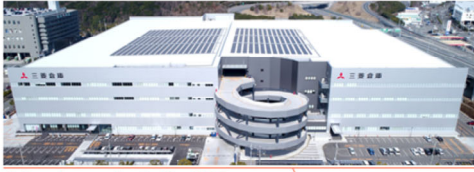
Full-scale operation in May 2020 Warehouse area: 36,342 m 2
