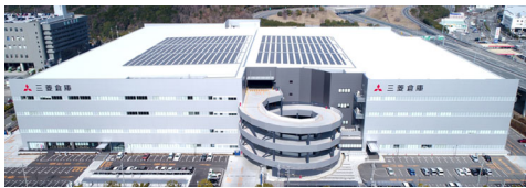
Full-scale operation in May 2020 Warehouse area: 36,342 m 2
