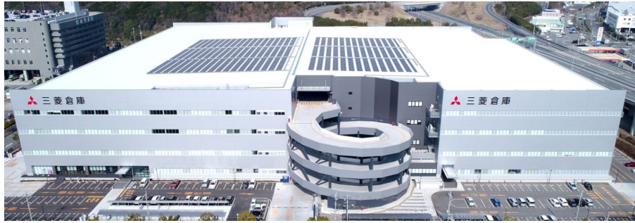
Full-scale operation in May 2020
